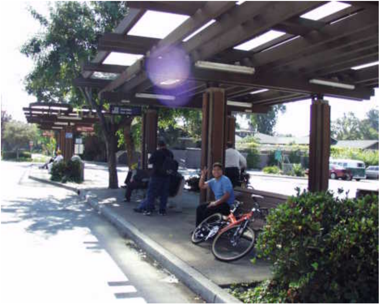
Figure 3 Palo Alto Caltrain Station Bus Shelter
