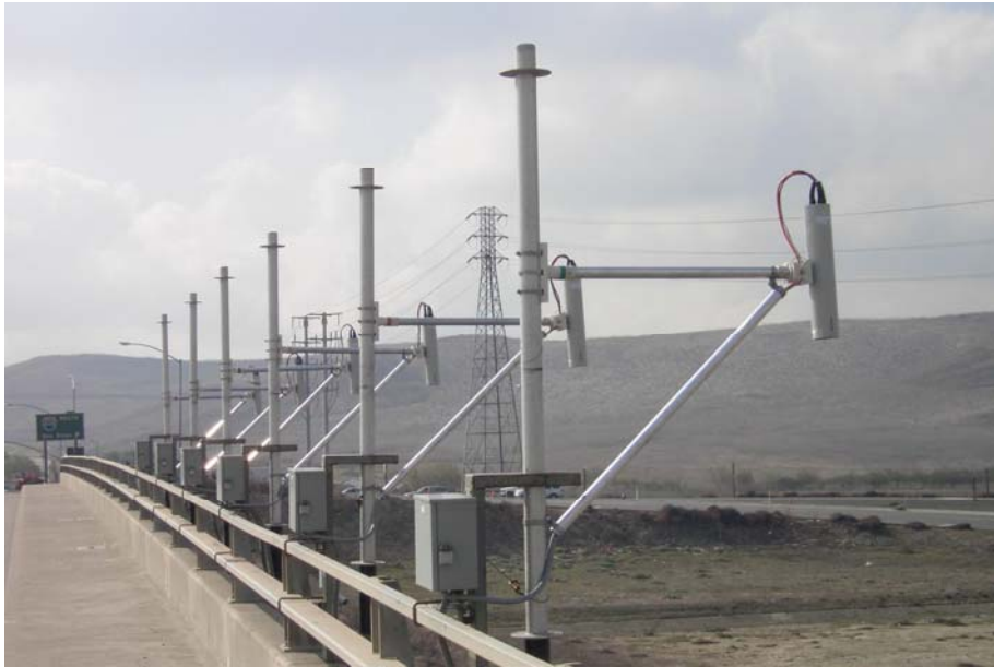
Figure 7.2. V2DVS cameras at Sand Canyon Test Site, showing proper camera positioning.
