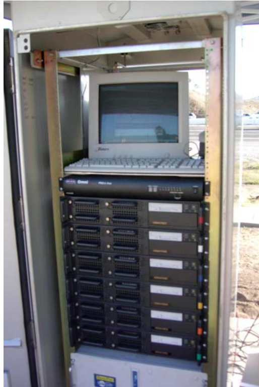
Figure 1.2 V2DVS Data Acquisition Computers in Type 334 Cabinet, Testbed Site at Sand Canyon Overcrossing.
