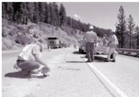
*Magnet installation on I-80 over Donner Pass. Top: Drilling holes for magnet placement. Bottom: Sealing holes after magnets have been placed.*
