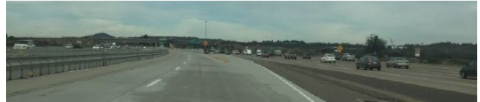
Fig 1. Ingress/Egress Section of I-15 Express Lane Facility.
