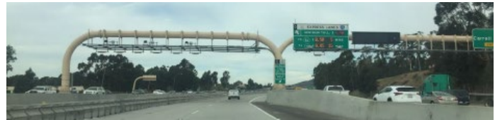
Figure 4. Changeable Message Signs on I-15 Express Lane.
